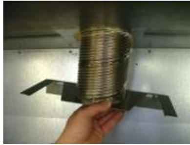
Push the spigot and liner back in place and secure the spigot via the 2 self tapping screws (see fig. 66)
