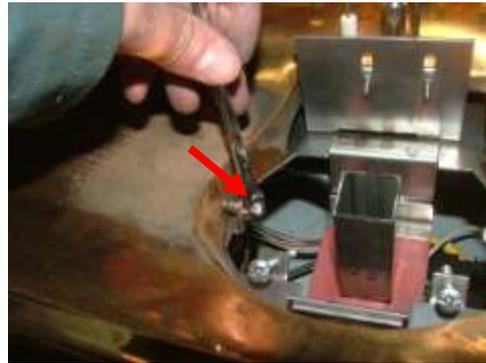
Before fitting the burner check the seal is in place. (Fig. 115)
