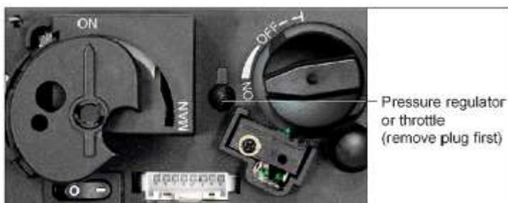
Fig.M6: Combination Control GV60, Cover
