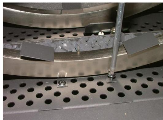
Place log 1 so that the knuckle is sat on the burner ridge, note the position of the log to the pilot. (See fig. 76)
