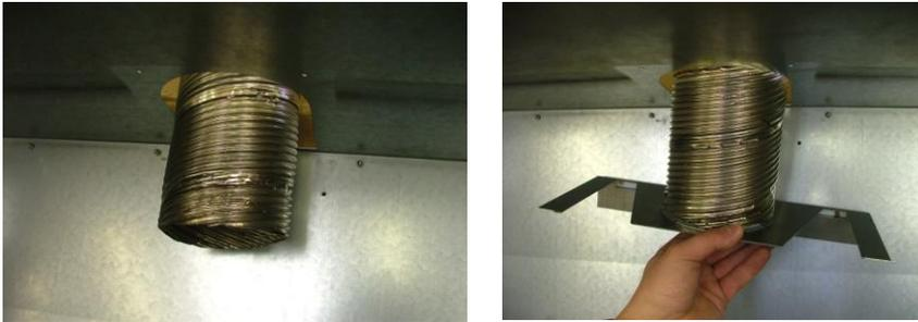
Push the spigot and liner back in place and secure the spigot via the 2 self tapping screws (see fig. 48). To ease the fitment of the inner casing the preferred gap between the spigot slide and top on the outer casing is 6mm (see fig. 49).
