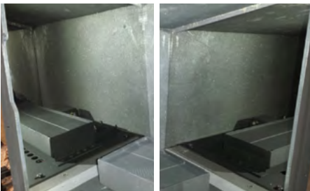
Fig.7 Stainless steel panels
